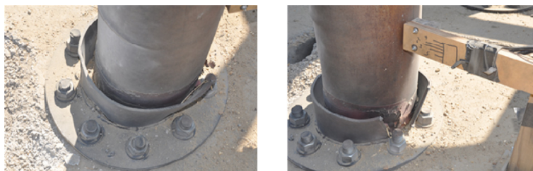
Fig. 13. Postshot failure of collar on Specimen MSJC2
