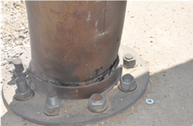
Fig. 8. Mark on steel jacket resulting from bearing on collar
