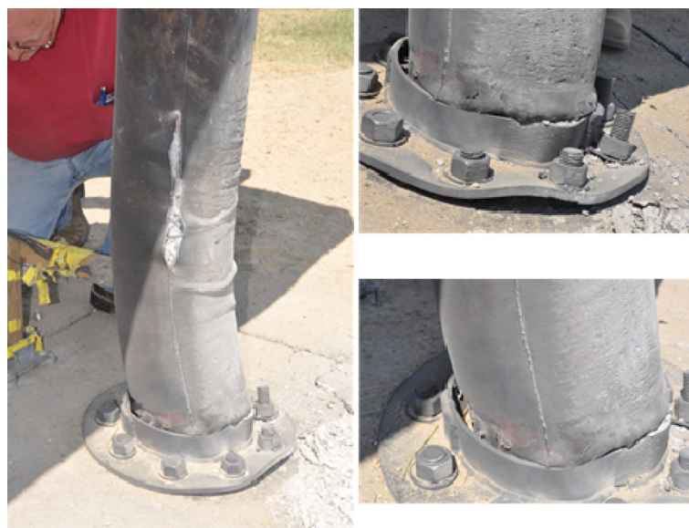
Fig. 7. Seam failure of Specimen MSJC1 and base deformation
